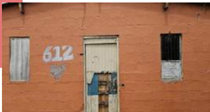
*Some of the houses before retrofitting
